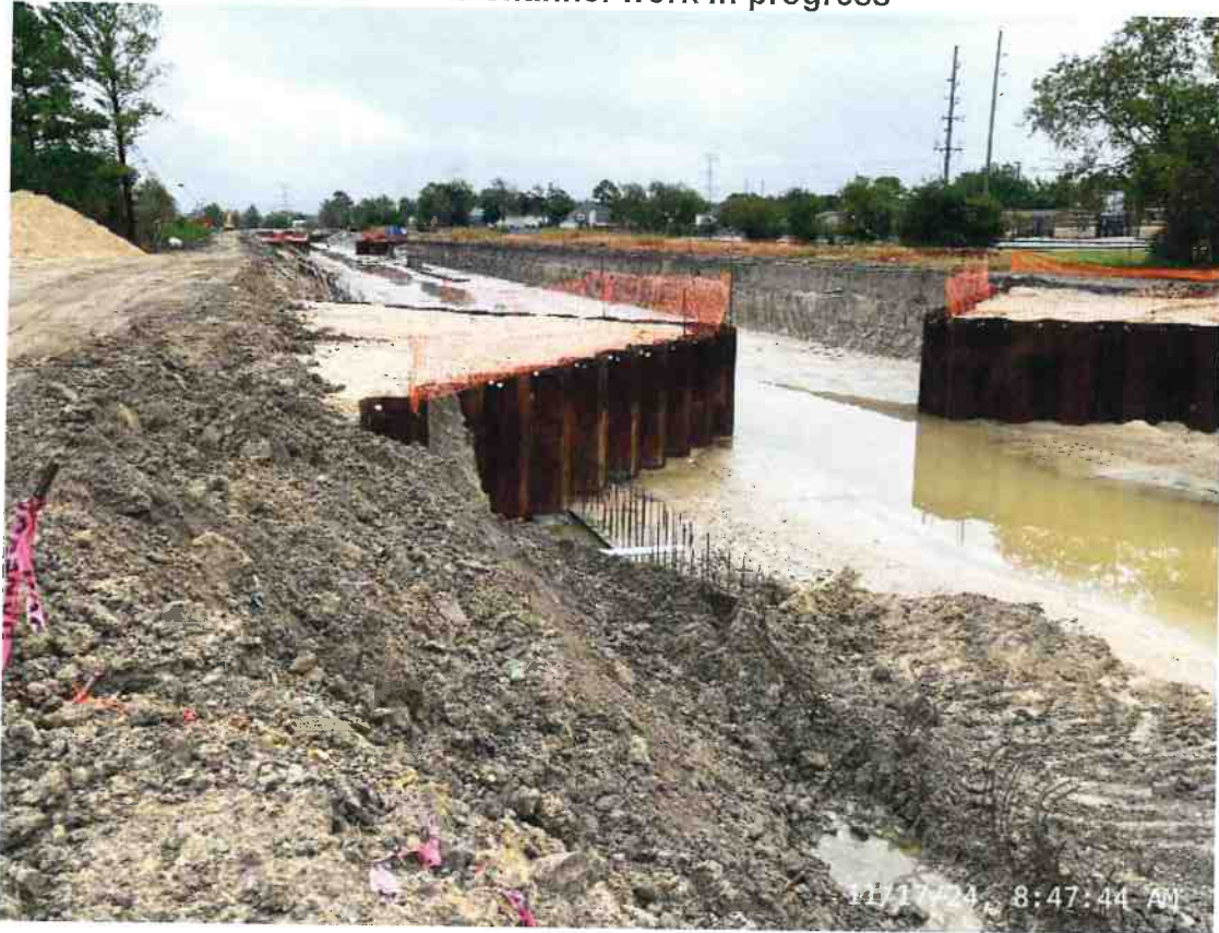
HCFC channel work in progress
